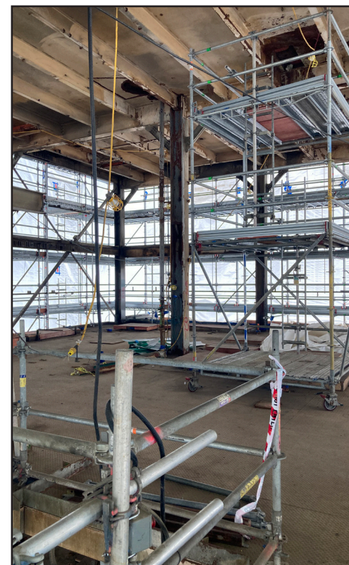
Left: Building 27 as it appears from the outside. Right: Building 27 on the inside. All exterior building panels have been removed revealing the structure of the building. The structure will be slowly dismantled over the rest of the year.
