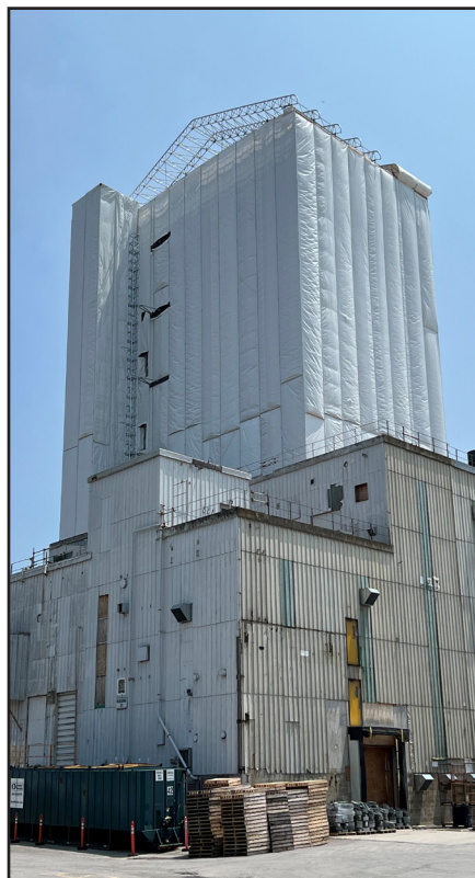
Left: Building 27 as it appears from the outside. Right: Building 27 on the inside. All exterior building panels have been removed revealing the structure of the building. The structure will be slowly dismantled over the rest of the year.
